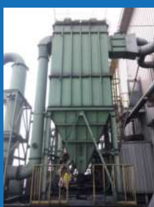
Return Carbon Tank
